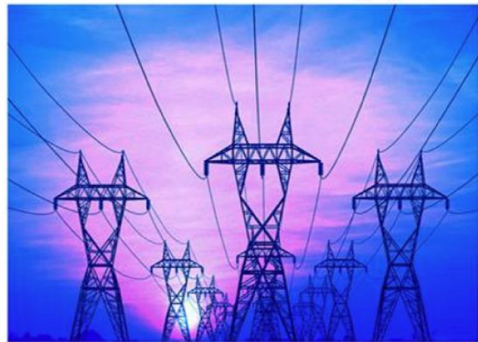
Performance Analysis of Hybrid Techniques for Evaluation of Power Transmission Cost and Loss Allocation Based with Transmission Reliability Margin
