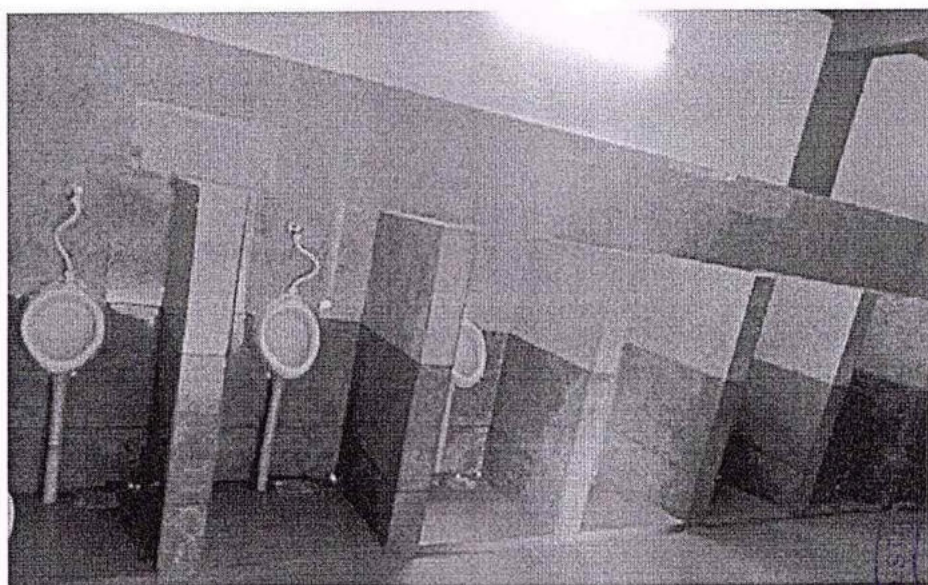
Western Toilets in Main block
