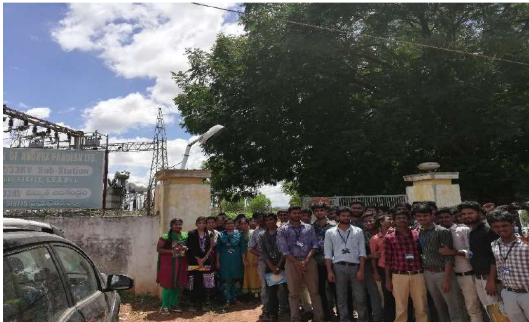
220 KV SUBSTATION BRAHMANAPALLI
